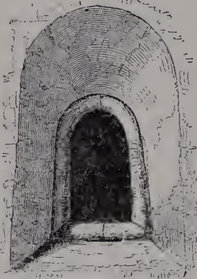
Anglo-Saxon Single-light Window, Tower of Wyckham Church, Berks.
